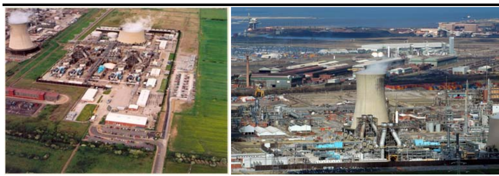
Figure 6.10 Former Teesside Power Station at the Project Site (now demolished)
