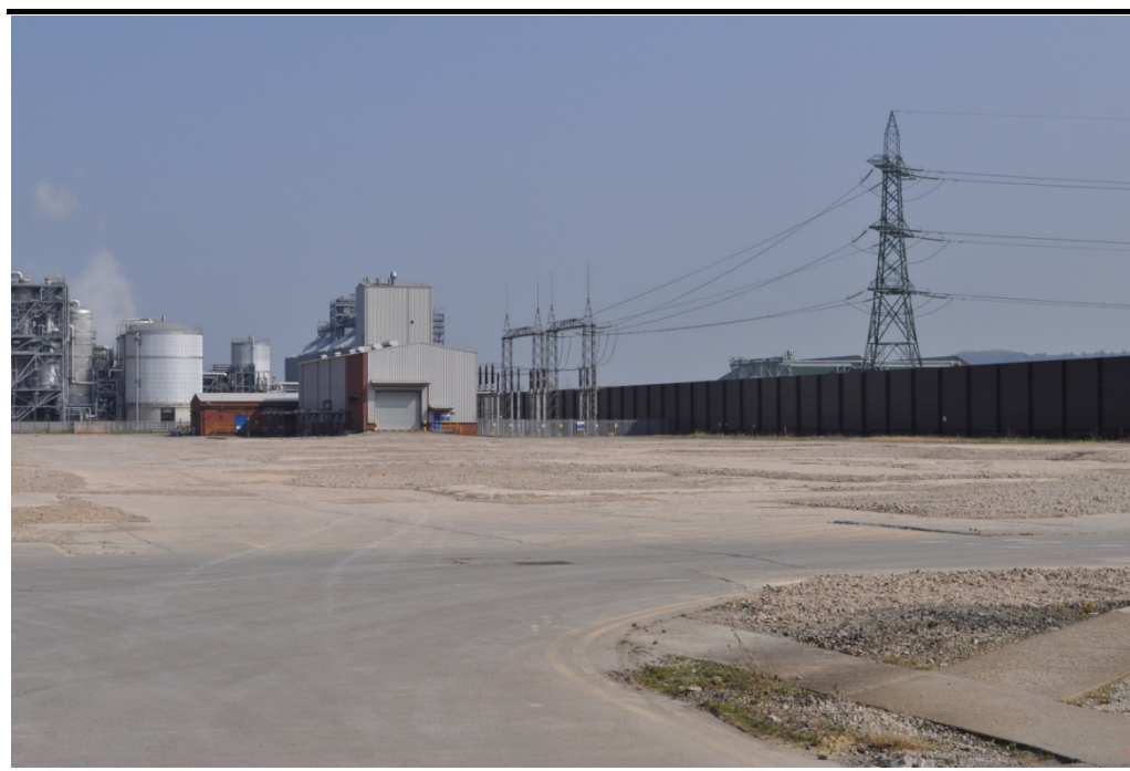
Figure 3.1 Existing Noise Control Wall
